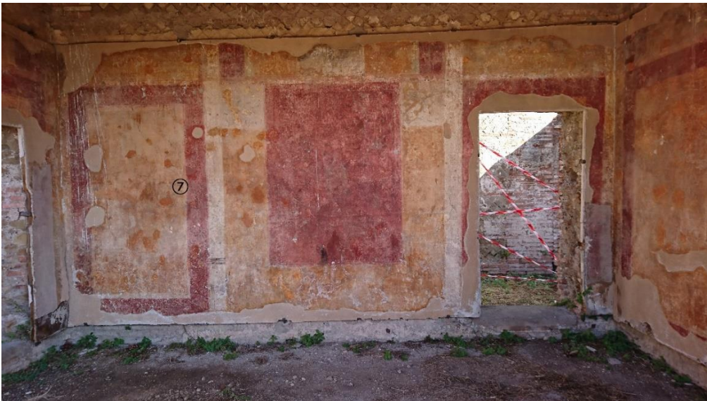
Fig.9 North wall of 13-4
