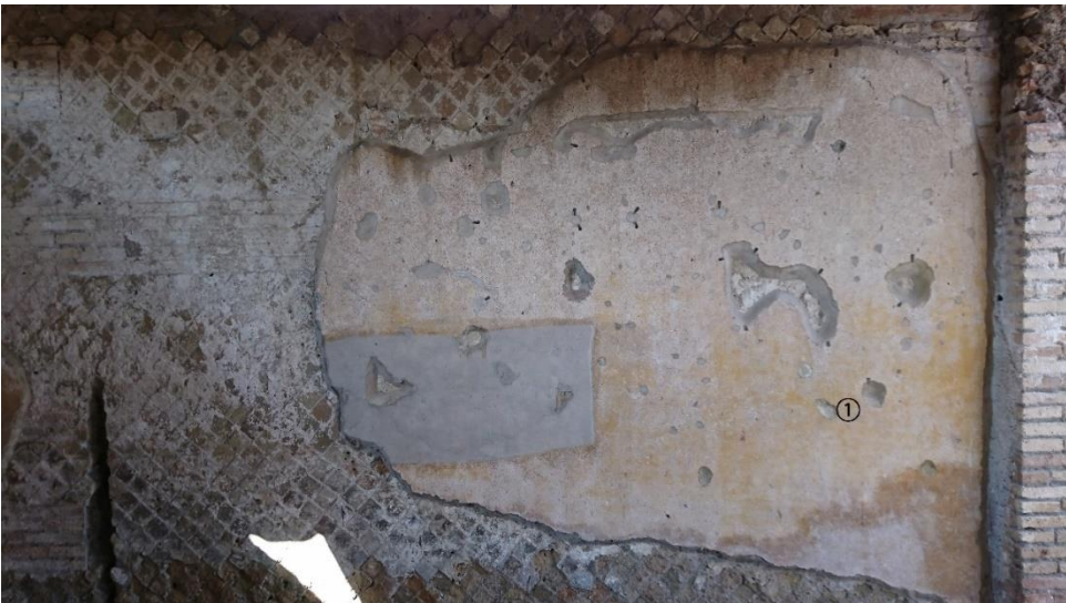
Fig.27 West wall of 20-7
