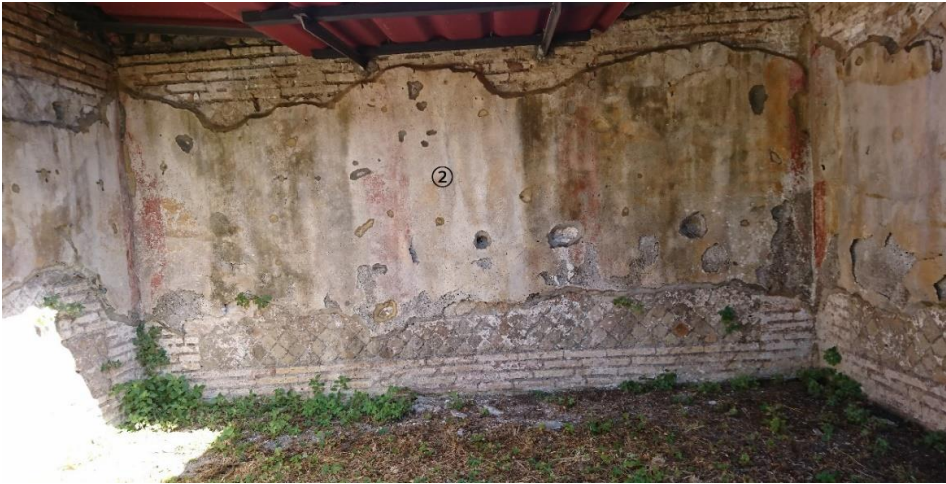
Fig.25 North wall of 17-7
