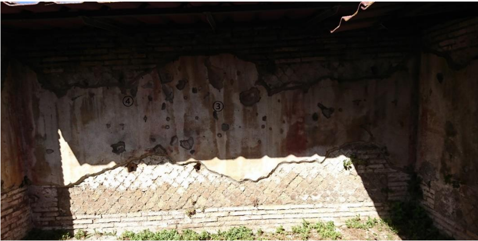
Fig.26 West wall of 17-7
