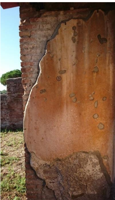
Fig.14 South wall of 15-7
