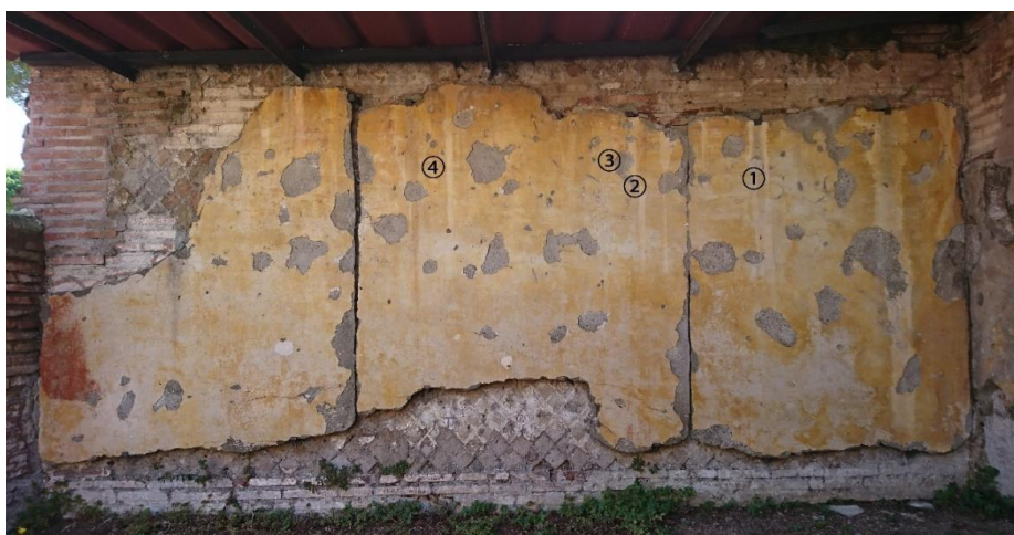
Fig.19 East wall of 16-7
