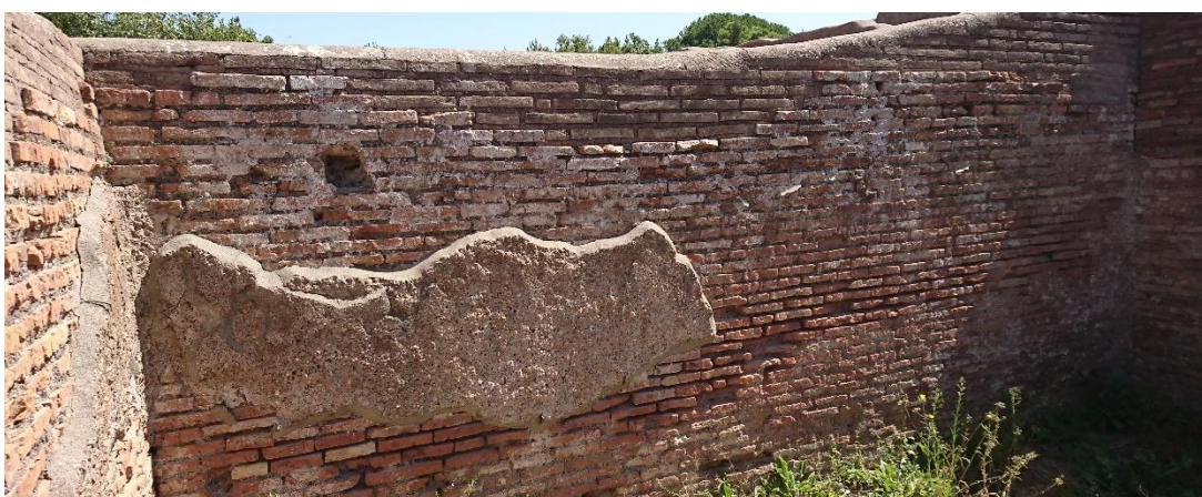
Fig.5 Bricks and plaster
