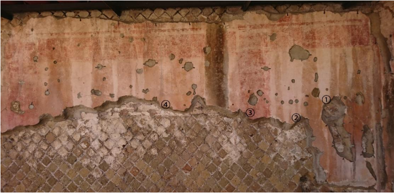
Fig.13 East wall of 14-5
