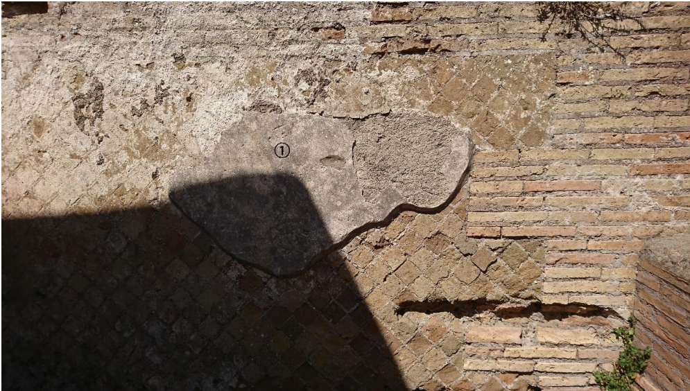
Fig.20 West wall of 17-1
