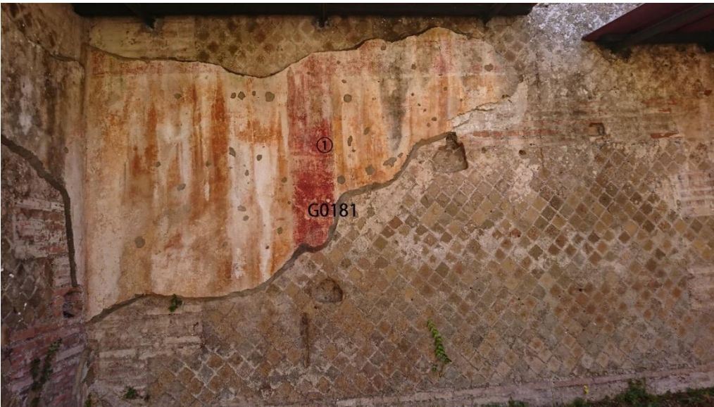
Fig.11 East wall of 13-5
