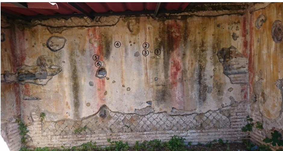
Fig.23 North wall of 17-6
