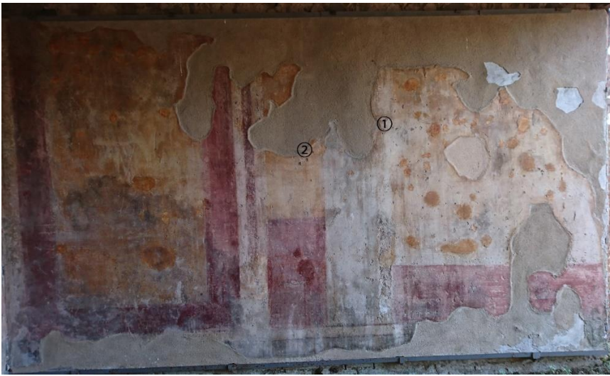
Fig.16 West wall of 16-5
