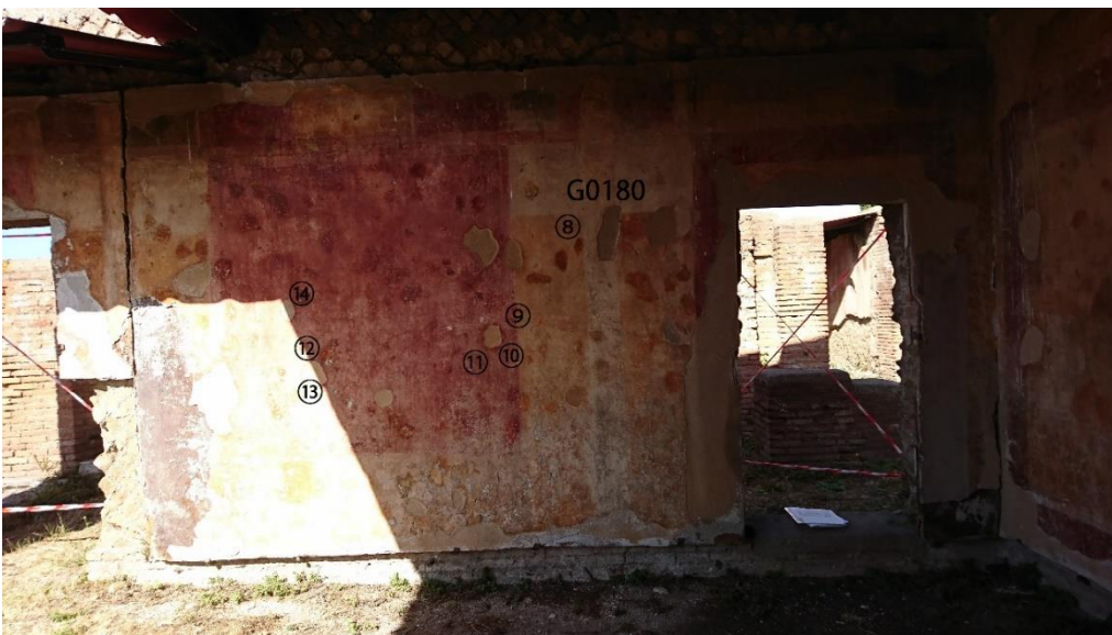
Fig.10 West wall of 13-4
