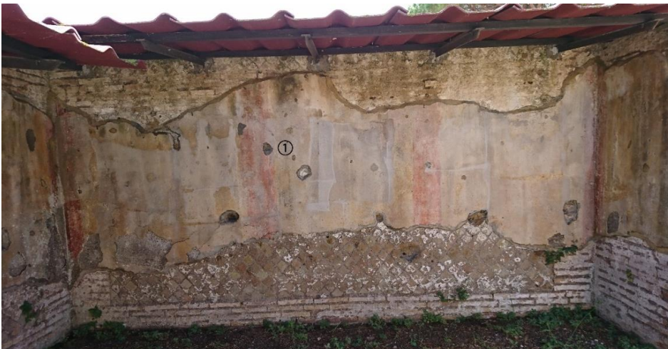
Fig.24 East wall of 17-7
